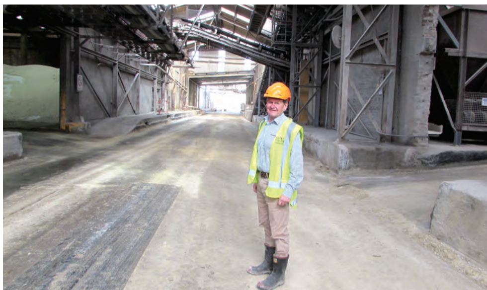
Ravensdown regional manager Mike Davey in the former meatworks, which has been home to Ravensdown in New Plymouth and before that New Zealand Farmers Fertilisers.
