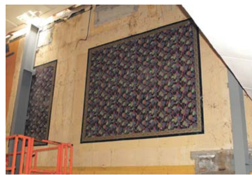
In the interior of the auditorium of the historic Everybody's Theatre these decorative feature walls were discovered when the cladding was removed. Hopefully they can be preserved. The reinforcing beams are visible either side.
