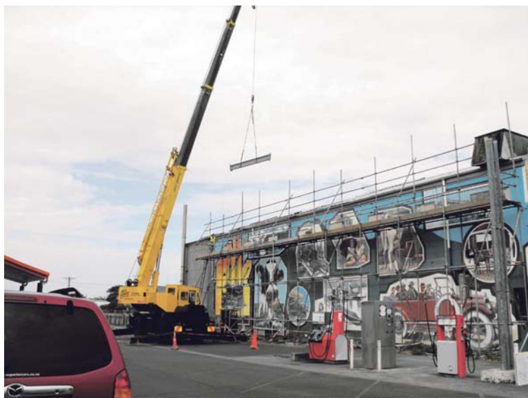
Lowering the reinforcing beams into the theatre via the roof.
