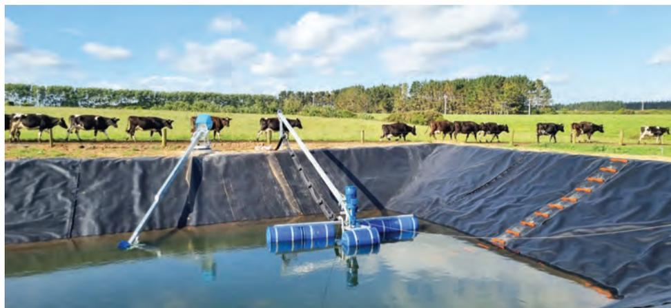
An Electric Stirrer Pondboom Centrifugal Pump-lined pond.
