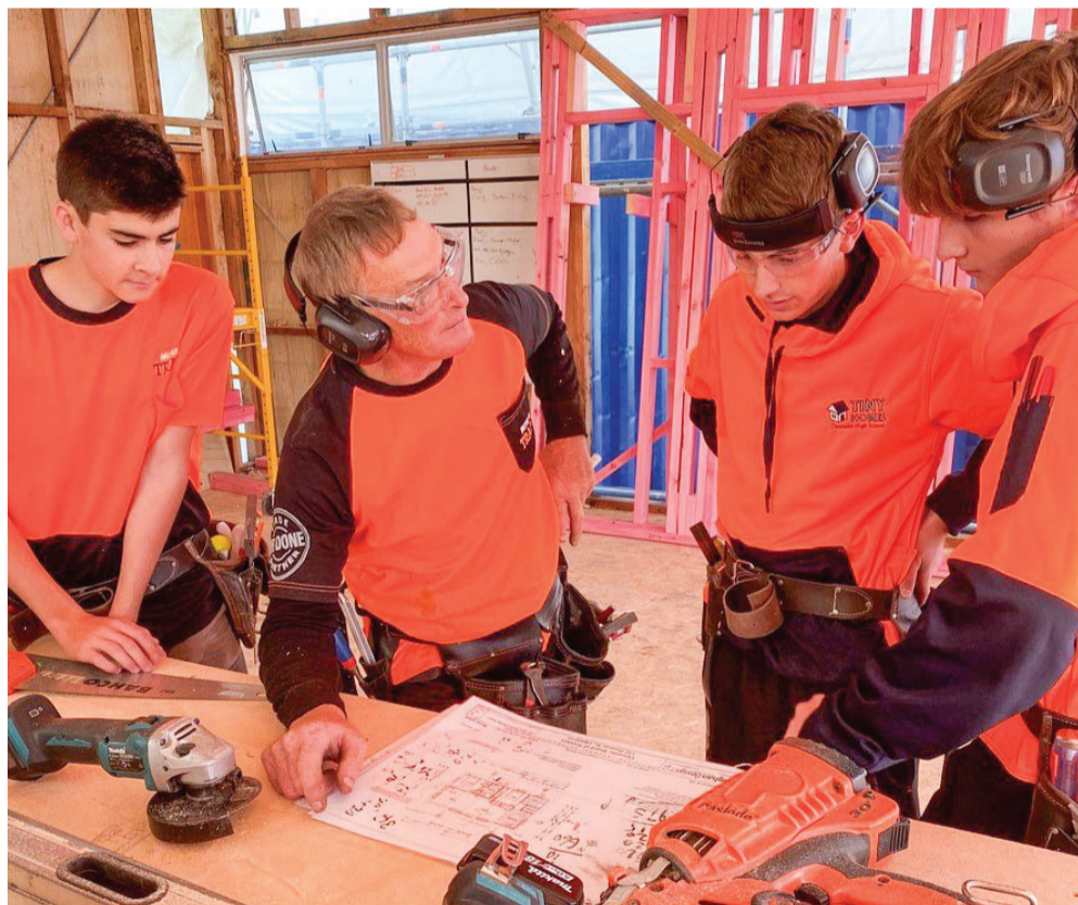
From left Ryan Buhler, Phil Hooper, Connor Forsyth, and Caleb Pattison. looking at plans of the intended building work.
