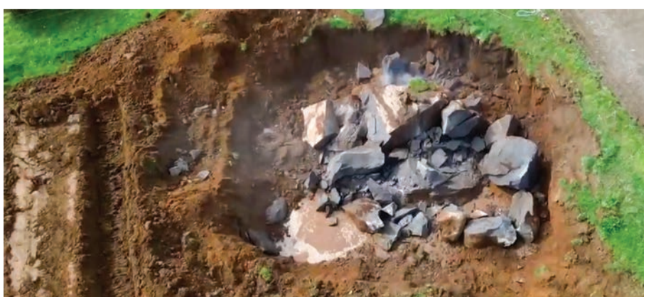
The end result, the rock blown into manageable pieces which were subsequently buried.
