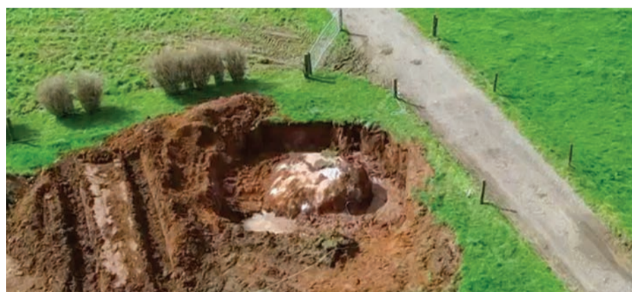
The large rock which has been exposed by digging a trench around it.
